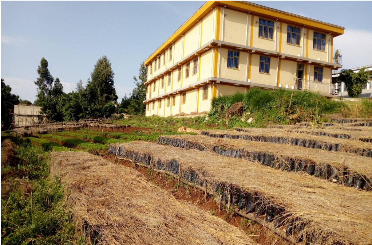
Figure 18. Photos of marvellous building of Bedele ARC and land owned by the center
