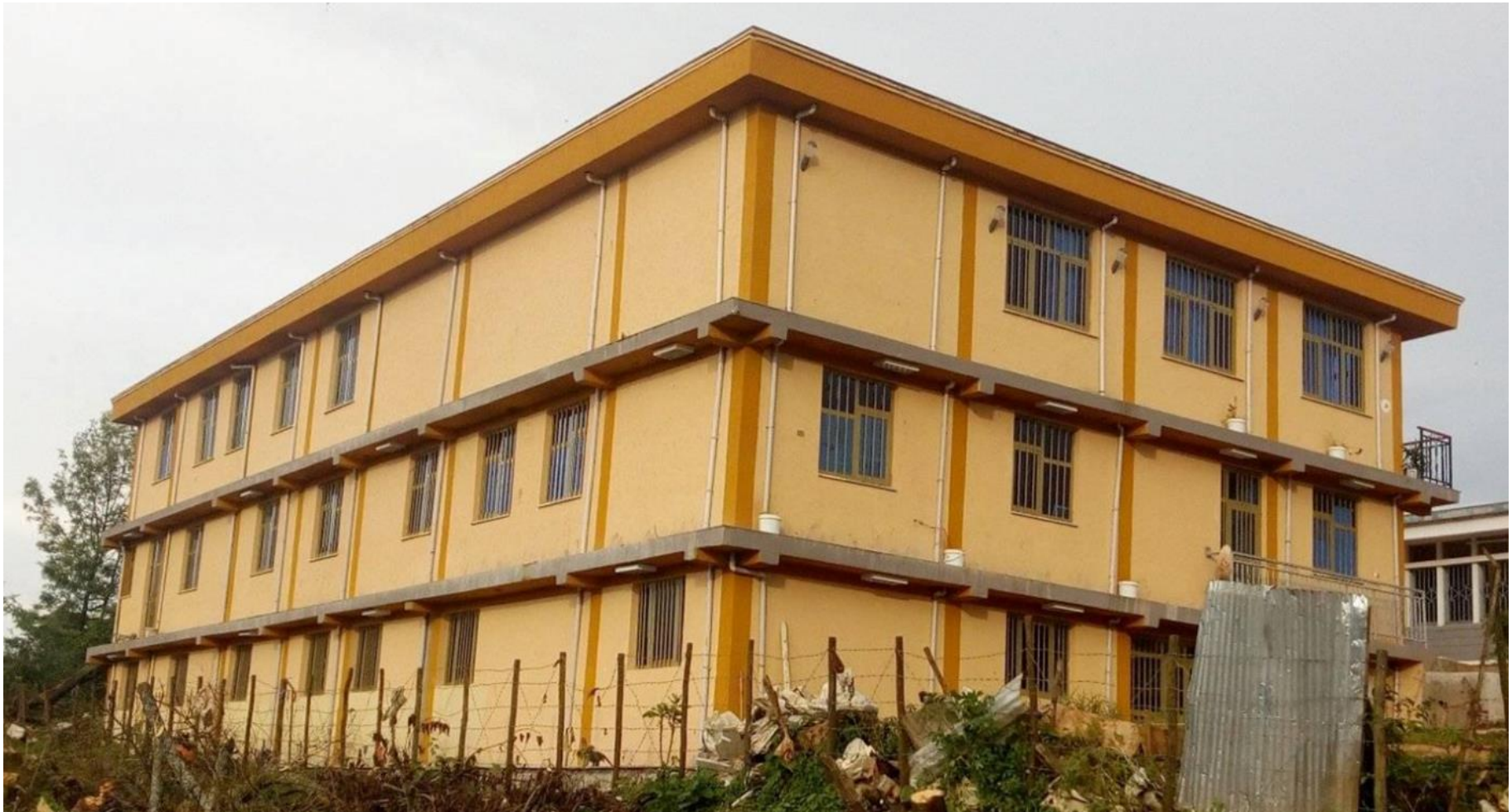
Figure: Marvellous building of Bedele ARC (supported by AGP-II)
