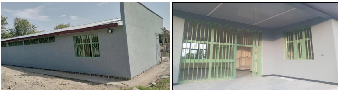
Fig 19. Status of Indoor hatchery building construction done on 300m 2
