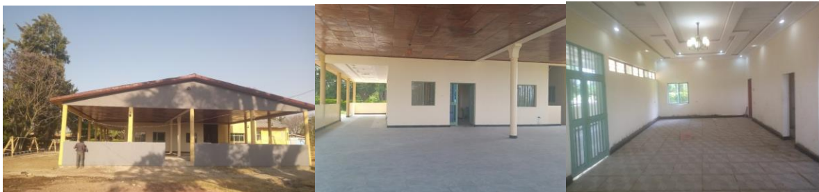
Fig 18. Status of Cafeteria construction status on 450m 2
