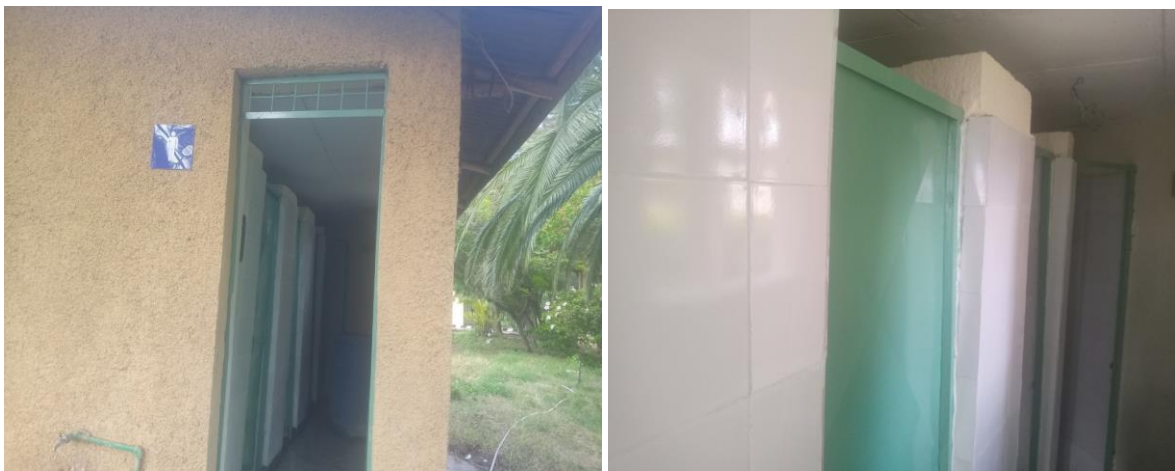
Fig 20. Status of Maintenance of old toilet were done (8 rooms)
