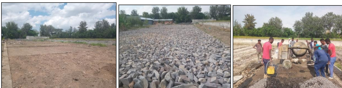
Fig 21. Status of Outdoor hatchery pond construct on 952m 2 (under construction)
