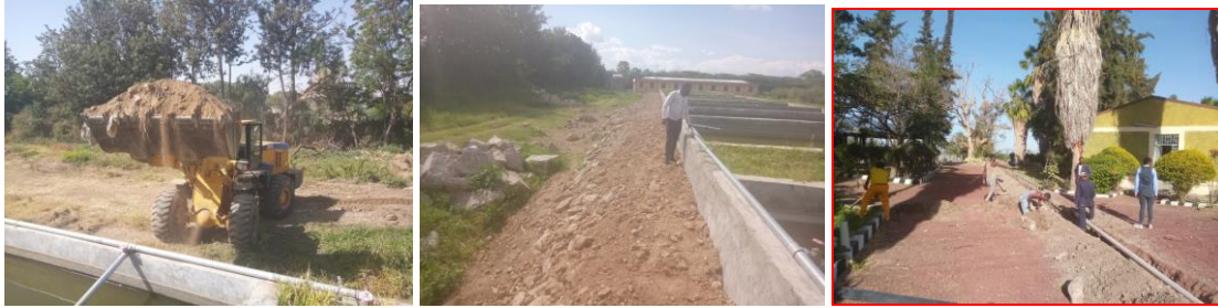
Fig 20. Status of fish pond area maintenance
