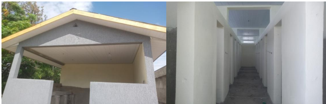
Fig 17. Status of Bath (10), Rest (10) & Washing Rooms (2) (supported by AGP-II)
